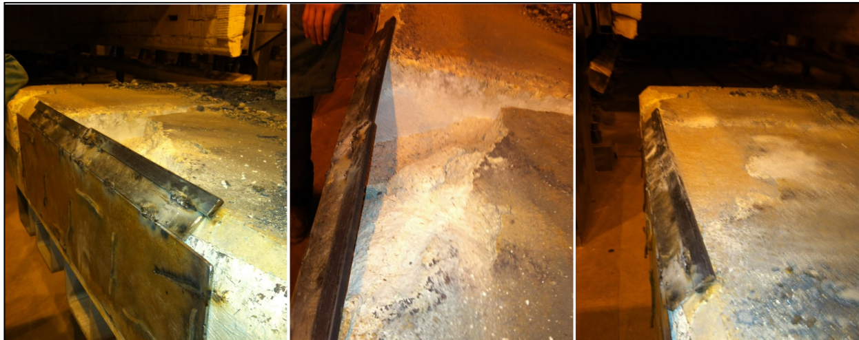
QUICK-FIRE® 65 perimeter repair
