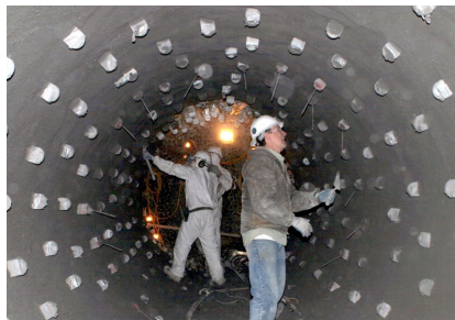
TUFFCRETE® 65 M shotcreted in rotary kiln
