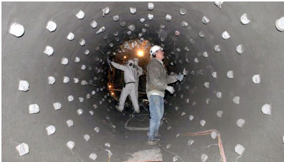
TUFFCRETE® 65 M SHOTCRETED CHAIN SECTION
