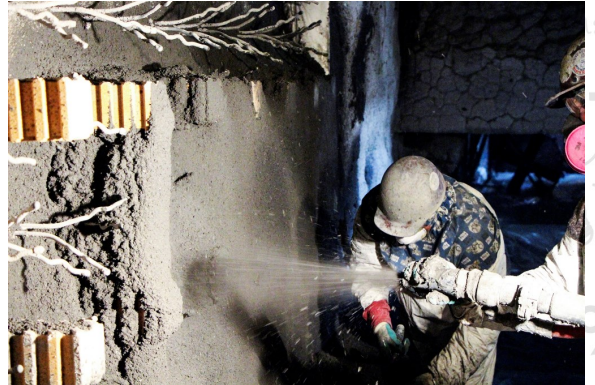
TUFFCRETE® 60 Z SHOTCRETE COOLER WALL
