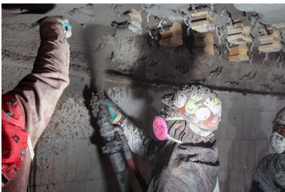
TUFFCRETE® 60 X SHOTCRETED CYCLONE ROOF
