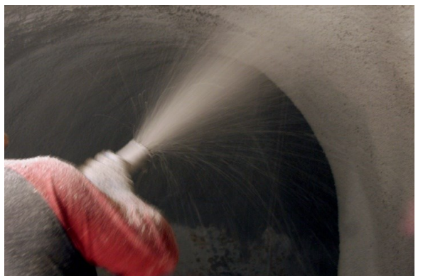
TUFFCRETE® FUSED SILICA SHOTCRETED DUCT
