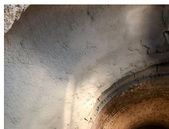
Firing hood flashed with QUICK-FIRE® 60 G
