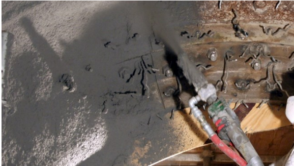
TUFFCRETE® 70 ABR SHOTCRETED TAIL RING
