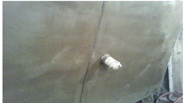
TUFFCRETE® SHOTCRETE SURFACE TROWELLED SMOOTH
