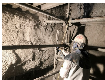
Cooler flashed with QUICK-FIRE® 60 G
