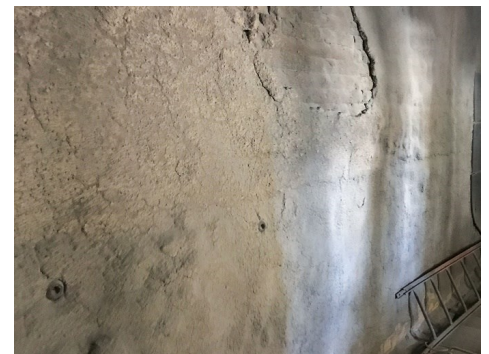
Cooler flashed with NANO-TEK® 60ZG. Majority still in place after 9 months of service.
