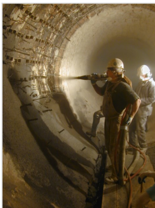
Shotcrete Installation
