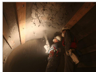
Shotcrete Installation
