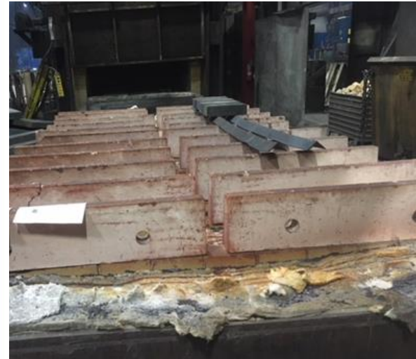
ARMORMAX® 70 SR pier blocks after 2 years of continuous service
