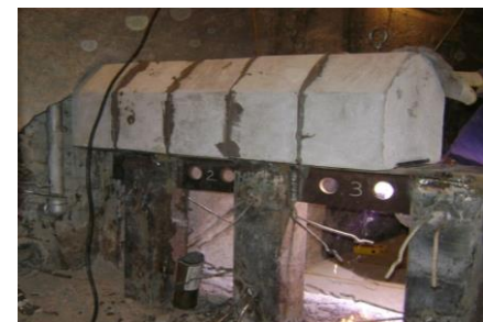
Cricket wall installation
