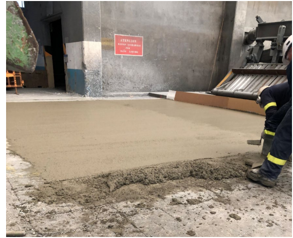
TUFFLOOR® after casting
